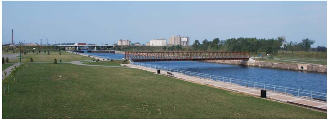
Complete brownfield remediation at Buffalo Lakeside Commerce Park
