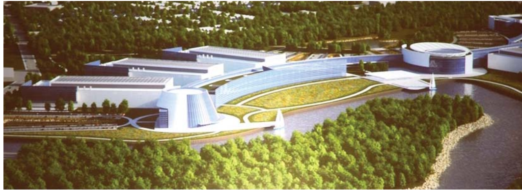
Buffalo High-Tech Manufacturing Innovation Hub at RiverBend
