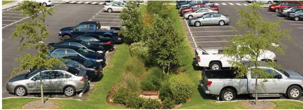
Image 21: Storm water mitigation using rain gardens
