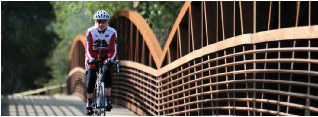
Image 49: Pedestrian bridge over river
