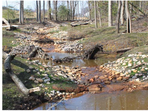
Image 56: Example of newly constructed Regenerative Stormwater Conveyance (RSC)
