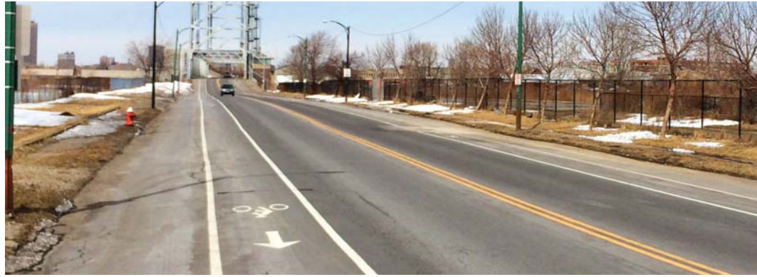
Image 19: Complete Street Infrastructure at South Park Avenue
