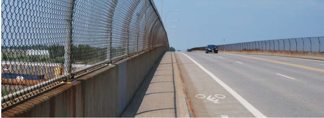
Image 27: Existing conditions on Tift Street Bridge
