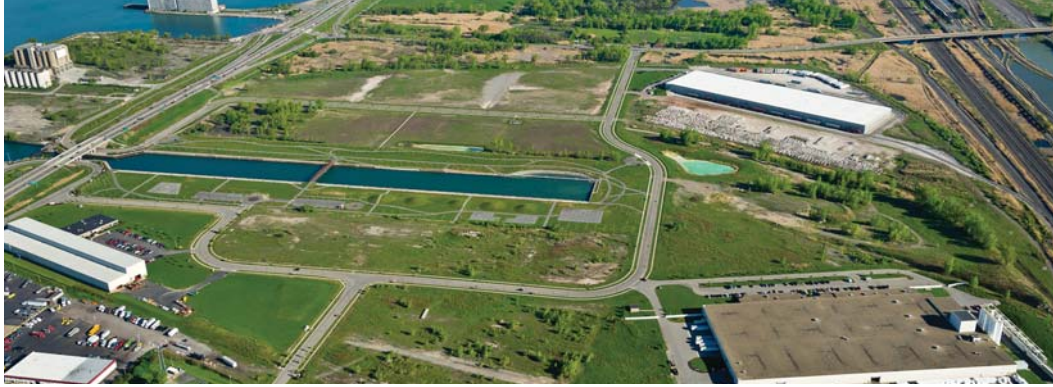
Image 35: Buffalo Lakeside Commerce Park Aerial
